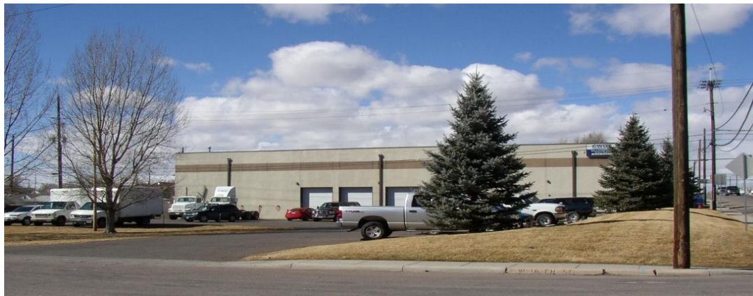
Manufacturing Facility and Shipping Warehouse, Cheyenne, WY
